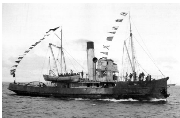
Fig. 3. The cutter Yelcho , owned by the Chilean Government, built in 1906 of steel construction. Her tonnage was 219 tons, displacement 467 tons, length 37 m and power 350 hp.
