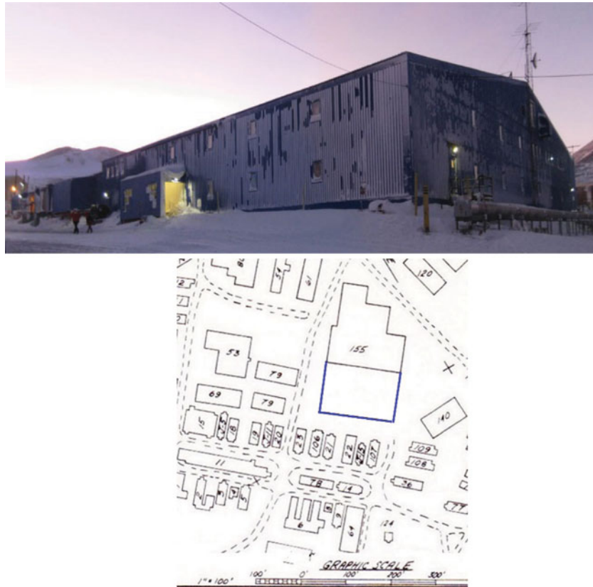
Fig. 13. (Top) Building 155, now painted blue, after a wind event, August 2010. Photo by author, 2010. (Bottom) Layout of Station around 1968 showing a half-built Building 155 (blue lines, added by author, show final extent) (USN 1968: 24).
