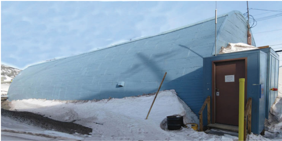
Fig. 9. A Quonset hut in McMurdo Station with a vestibule entrance addition. Photo by author, 2009.
