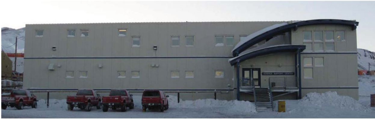
Fig. 15. The Science Support Center (SSC) built in 2004 (Photo by author, 2009).
