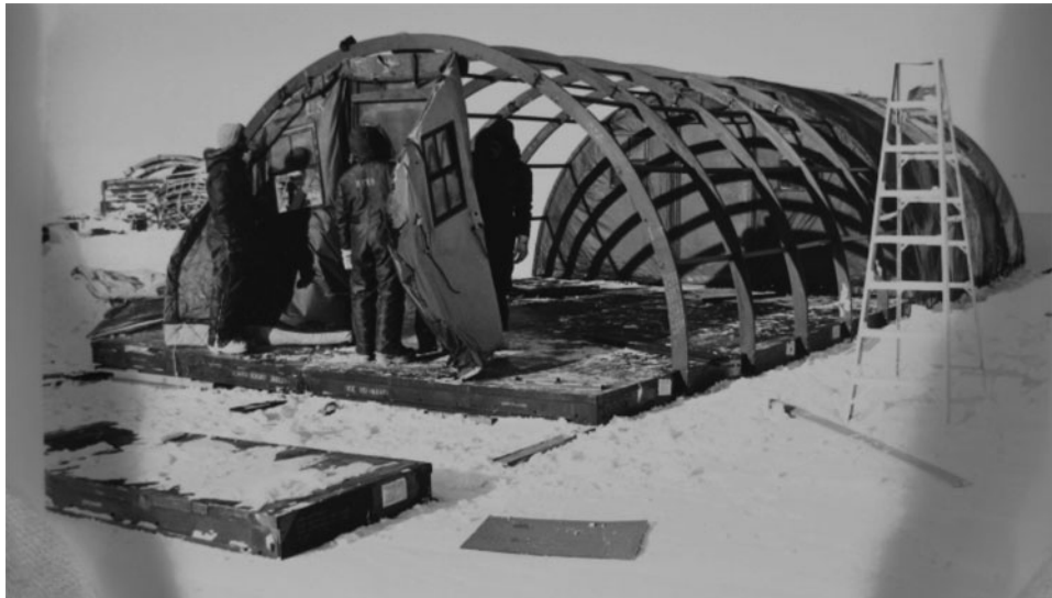
Fig. 10. Byrd Surface Camp, Antarctica. Jamesway tent under construction during the Deep Freeze 1980 season. (Note the flooring.) Photographer: Jeff Hilton. Date: Nov. 6, 1979. Naval Photographic Center, Naval District, Washington, D.C. Official U.S. Navy Photograph.
