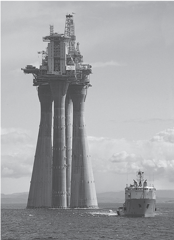
Figure 1.3 The Troll GBS under tow (courtesy Equinor).
