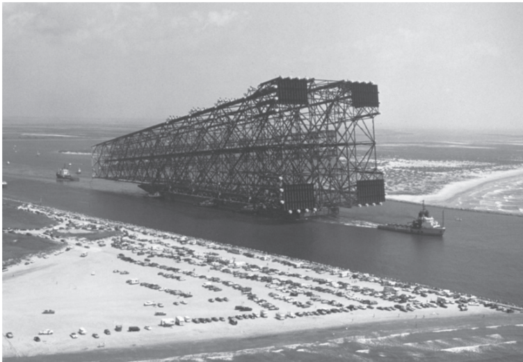
Figure 1.2 Bullwinkle jacket under tow (picture by Lanmon Aerial Photography, courtesy of Shell Exploration & Production Company).
