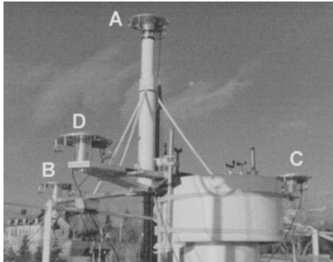
Figure 1. Antenna installation on board F. C. G. SMITH.
