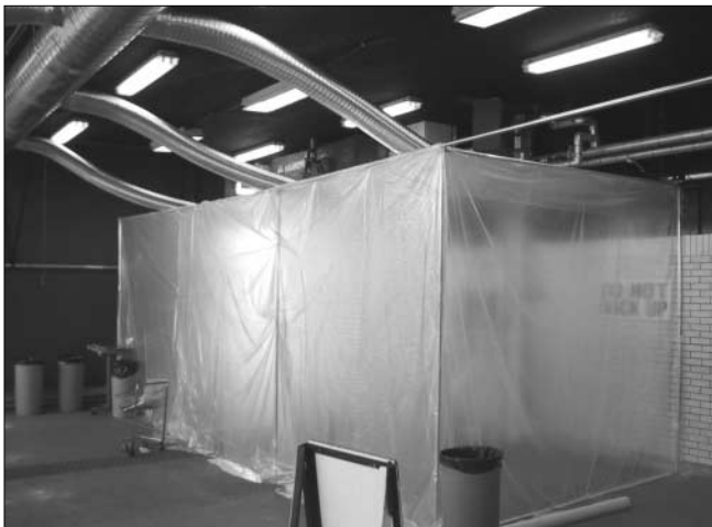
Fig. 2. Construction of examination rooms.
