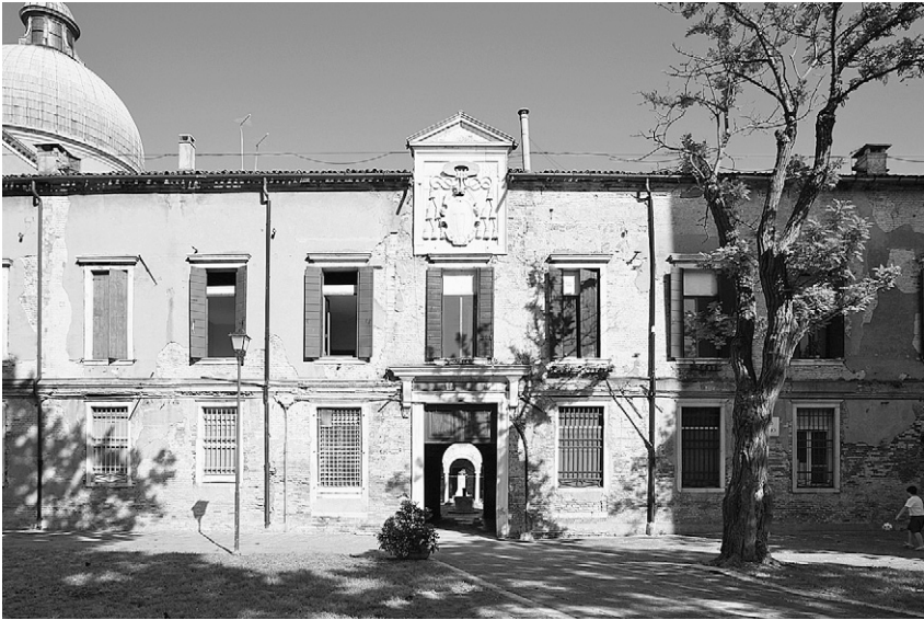
FIGURE 5. View of west façade, patriarchal palace, Campo di San Pietro di Castello, Venice. Photo: Seth C. Jayson.
