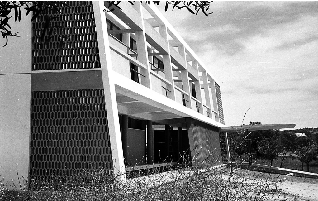
Fig. 4. The social service and childcare centre in Loulé, Portugal, Manuel Laginha and Rogério Martins, 1951–58, photograph of c. 1959 (DGPC/Forte de Sacavém, Arquivo Manuel Laginha)
