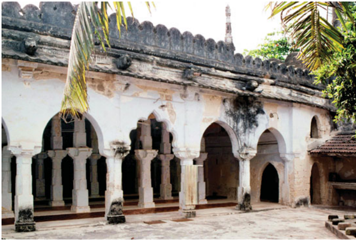
Figure 22. (Colour online) Idri's Masjid, view of the prayer hall from the south-east of the courtyard showing the arches added later to the façade, but otherwise the original colonnaded structure can be seen.
