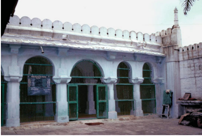
Figure 17. (Colour online) Chauḡān Masjid, view of the prayer hall from the courtyard looking north-west. Decorative arches on the façade of the prayer hall are later additions, but the original structure, such as the roof lintels and upper shafts of the columns, can still be seen on the surface.
