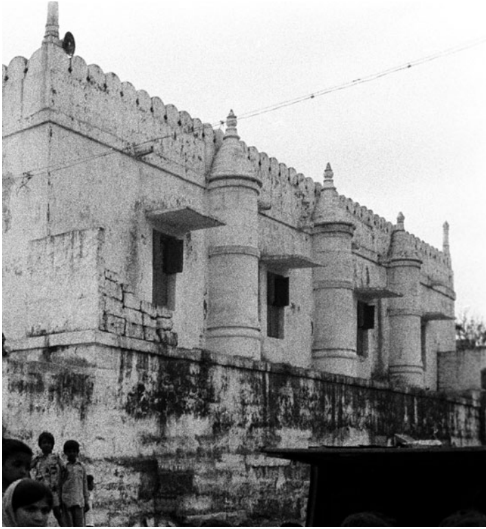
Figure 13. Somnath, Chauḡān Masjid, exterior of the qibla (western) wall of the prayer hall with its three projecting mihrābs standing over the high platform.
