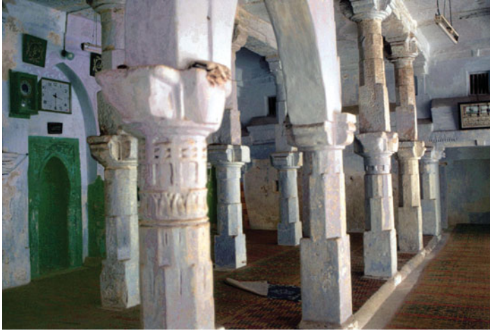
Figure 21. (Colour online) Idri's Masjid, prayer hall looking north-west and showing the central mihrāb and the general structure of the mosque with columns each composed of two shafts of similar size. The lower parts of the bases of the columns are now buried under the modern floor. The northern wall in the background is the walled-up northern gallery, where parts of the original parapet leaning out of the wall can still be seen.
