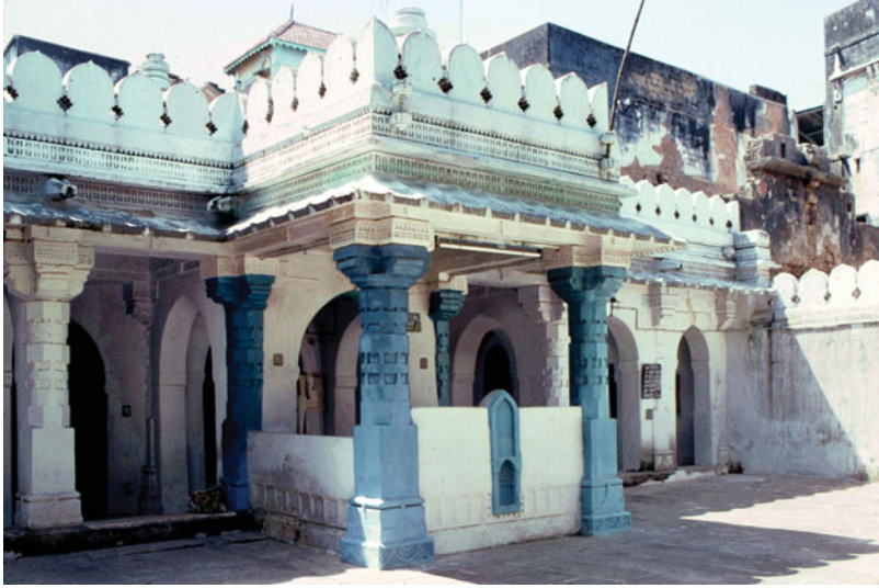
Figure 11. (Colour online) Mangrol, Chishtīwālā Masjid, view of the prayer hall from the courtyard looking north-west. The canopy attached to the front of the prayer hall was added later and contains a single grave which is said to belong to Khwāja Naṣīr al-dīn Kalān Chishtī. The arches between some columns in the prayer hall and the parapet around the tomb are also later additions.
