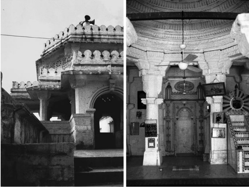
Figure 23. Una, the Jāmi' mosque. Left: the entrance chattrī ; right: the central bay of the prayer hall, showing the main mihrāb , and the domed unit of the central aisle with a finely decorated corbelled dome supported by columns, each composed of a complete shaft below and the upper half of a shaft above. The elements are carefully chosen and matched together.
