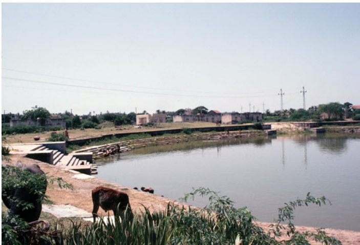
Figure 2. (Colour online) Bhal ka Talāo from the south-east, showing the southern steps at the far left and the western ramp, in a ruinous state, to the right. The stepped washing platforms around the reservoir are fairly well preserved and are still in use.
