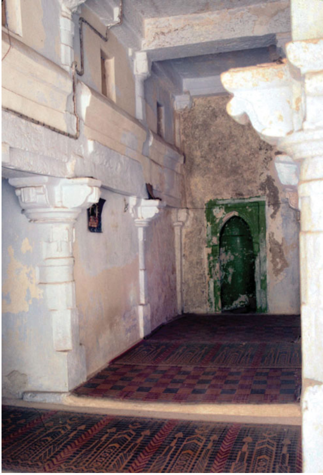
Figure 20. (Colour online) Idrīs Masjid, view of the southern end of the prayer hall, showing the southern mihṛāb and the walled-up mezzanine gallery supported by columns at ground level, also partly walled up. The parapets of the mezzanine can be seen projecting from the secondary walls. Much of the original decoration is covered by whitewash.
