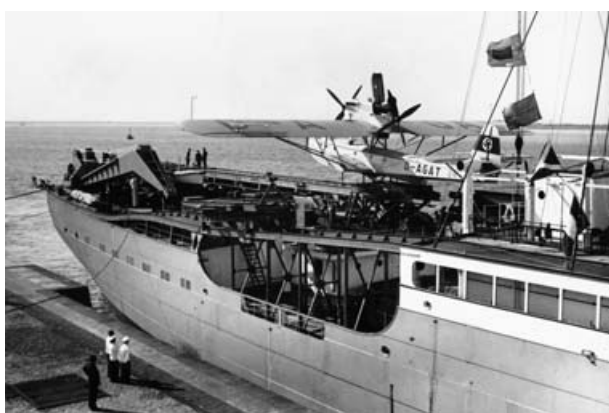
Fig. 3. Boreas flying boat on Schwabenland 's catapault (Courtesy Lufthansa).
