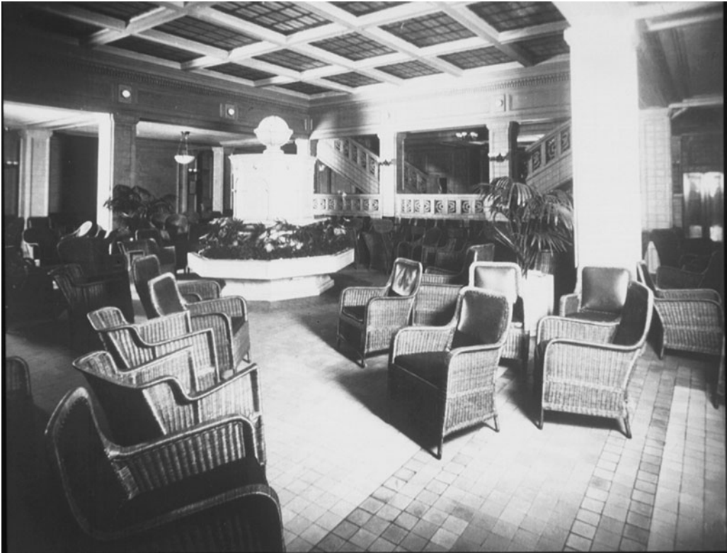
Figure 4. The fountain in the clinic lobby served both aesthetic and mechanical purposes. The building's air was tempered by running it through the fountain's heated (in winter) or cooled (in summer) water. Reproduced from Richard Olding Beard, "The Mayo Clinic Building, Rochester, Minnesota" Journal-Lancet , 34, no. 16 (1914): 428. Courtesy of the Minnesota Medical Society
