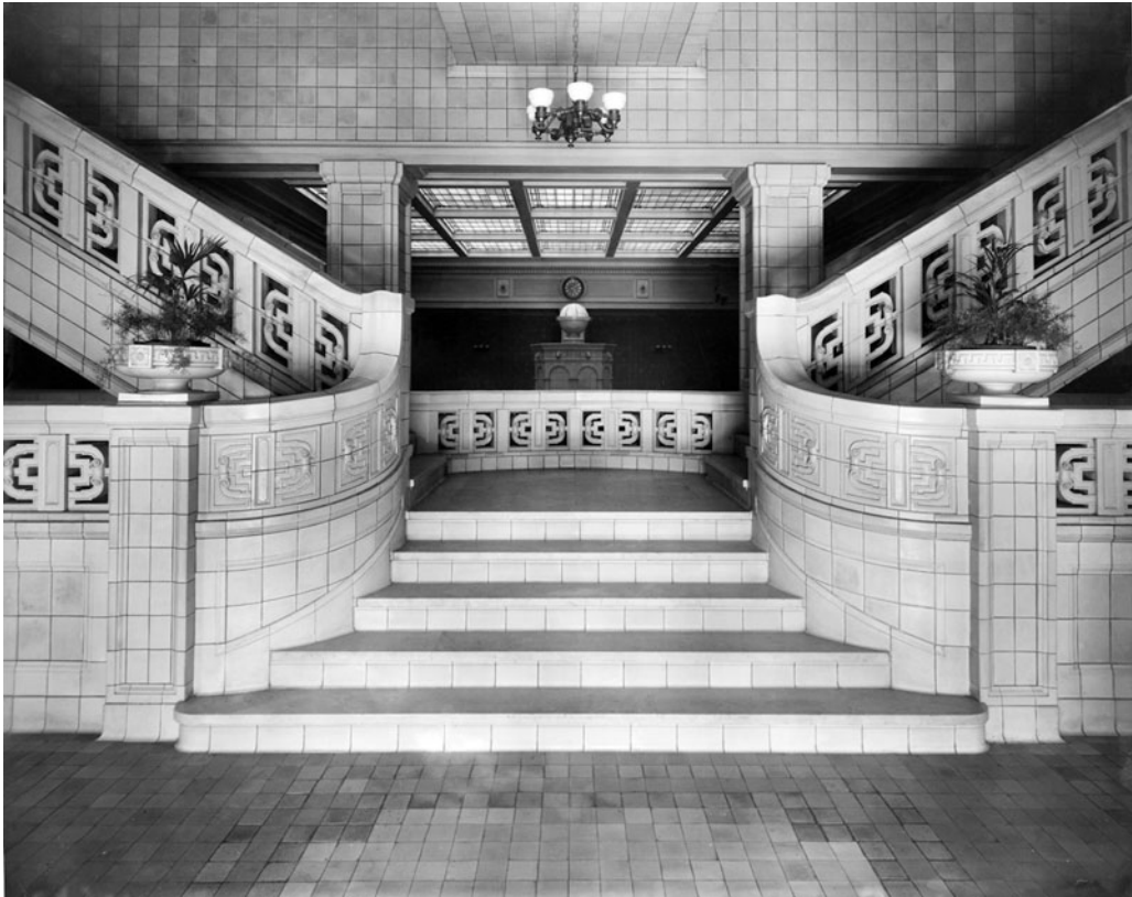
Figure 3. The building's central staircase. In general, the choreography of the building dictated that patients ascend by the right hand stairs only, while the left hand were for those who had already been processed and were on their way down. Reproduced from Richard Olding Beard, "The Mayo Clinic Building, Rochester, Minnesota" Journal-Lancet , 34, no. 16 (1914): 427. Courtesy of the Minnesota Medical Society
