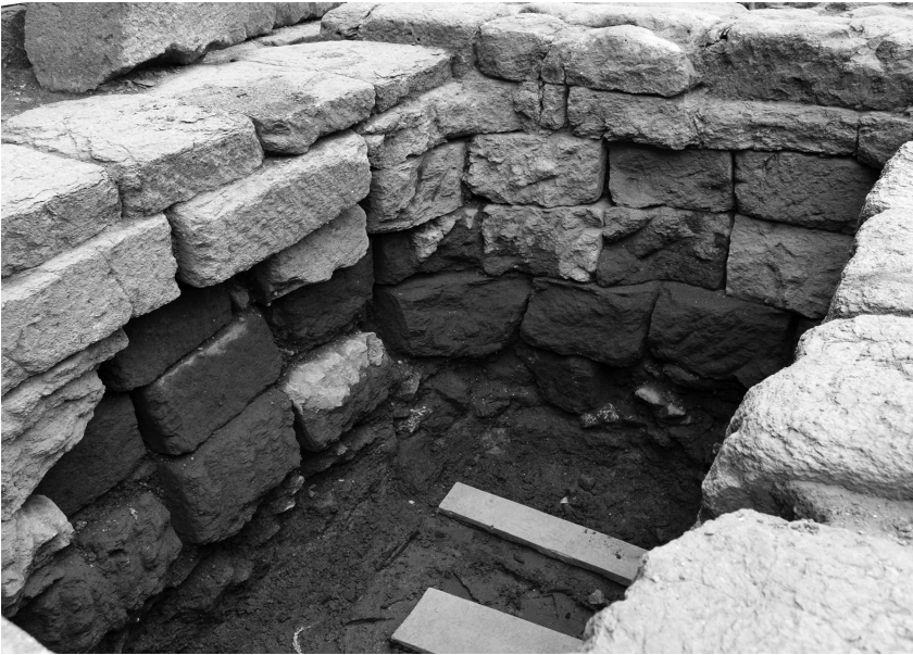
Fig. 5. Sounding D15 showing 6 courses of the Tufo del Palatino structure, looking southwest (D. Diffendale).
