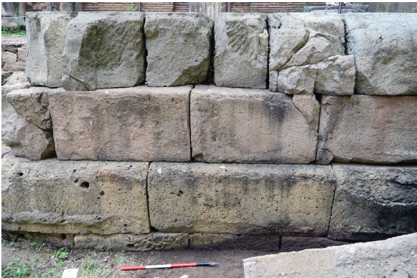
Fig. 16. N end of the E limit of the Republican podium, showing, from bottom to top, 2 courses of Tufo Giallo, 1 course of Tufo Lionato, and 1 course of Lapis Albanus, looking west (D. Diffendale).
