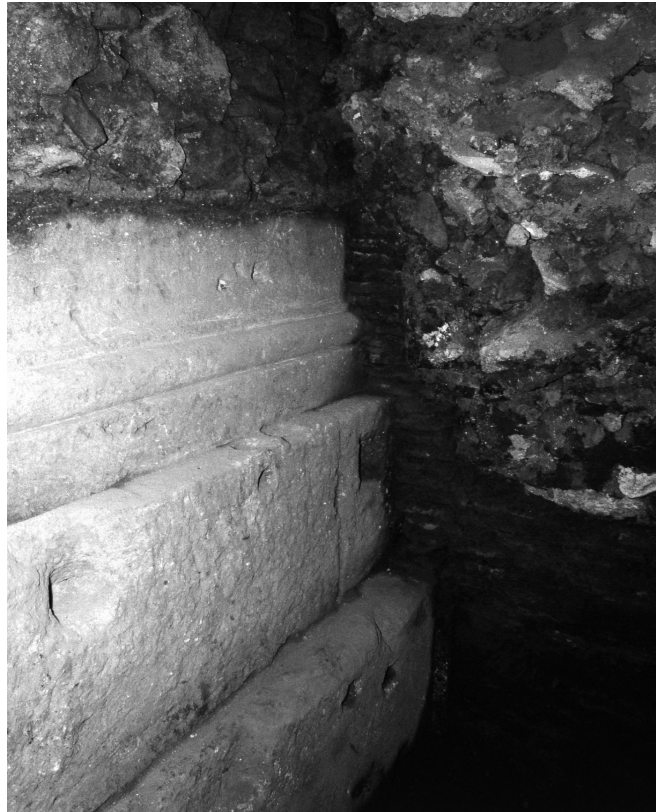
Fig. 17. Exterior of the N wall of the E cella , showing 3 courses of travertine, looking southwest (ASRCM).
