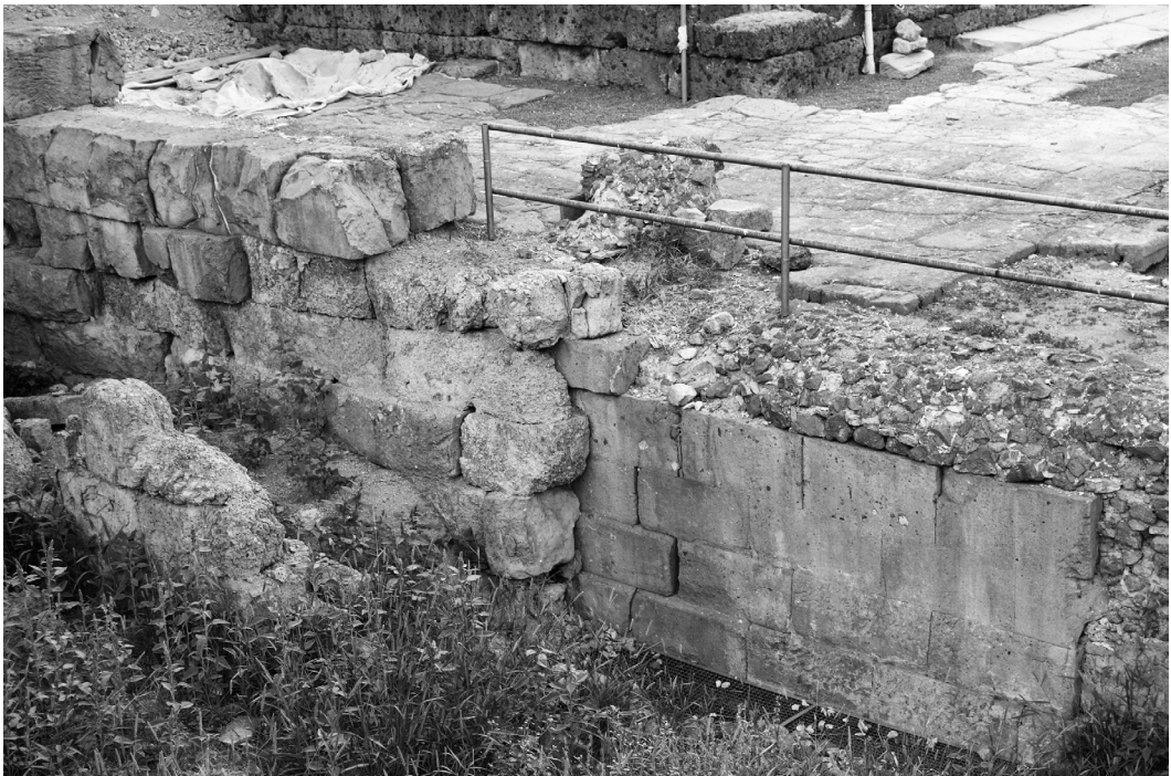
Fig. 8. W limit of the Republican podium, showing to the right 5 courses of Lapis Albanus; to the left 4 courses of Tufo Giallo, 1 course of Tufo Lionato, and 1 course of Lapis Albanus, looking northeast (D. Diffendale).
