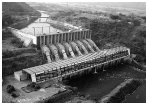
Figure 1. The 350 MW Inga Dam I in the DRC
