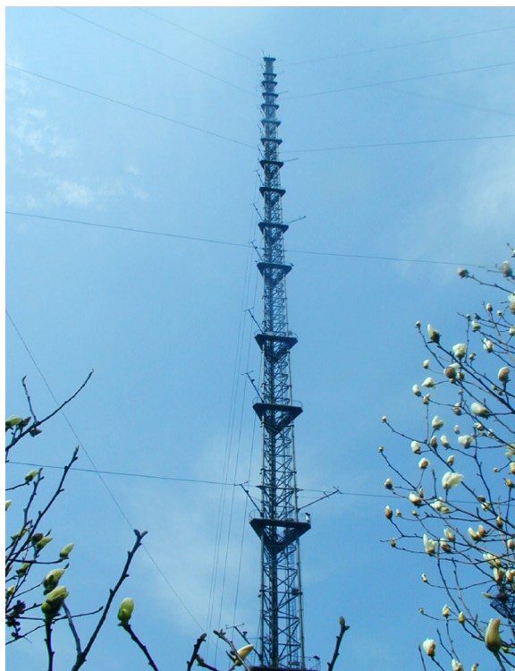
Figure 1. Observation tower employed by (Zeng et al. , 2010) to measure the vertical gradients in the urban boundary layer. This figure was taken from http://www.iap.ac.cn/xwzx/tpxw/201510/t20151010_4435945.html .
