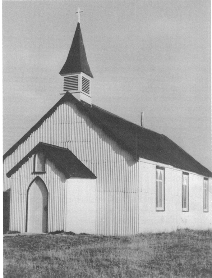
Fig. 12. Great Whale River, St Edmund's Church: constructed from a prefabricated kit in 1879 (Yellowknife, Northwest Territories Archives, Archibald Fleming Fonds, N-1979-050; 0298)
