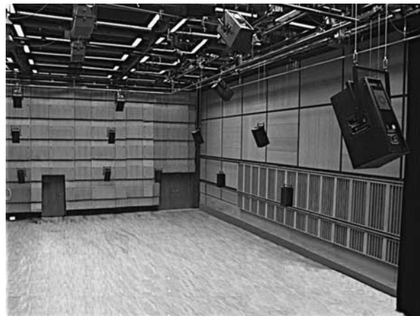
Figure 1. The Sound Dome in the ZKM's Cube theatre, with 47 loudspeakers. Photo: Bernhard Sturm © ZKM 2007.
