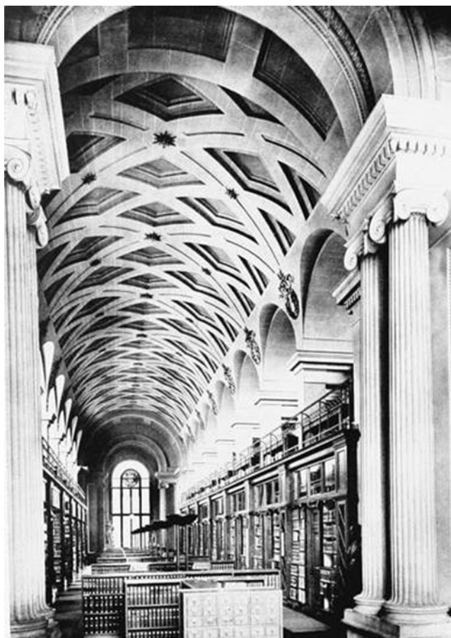
Figure 2. The first floor of the SLL in the Cockerell Building, Old Schools site. From ~1975 to 1995 Foreign & International Law materials were concentrated in this hall.
