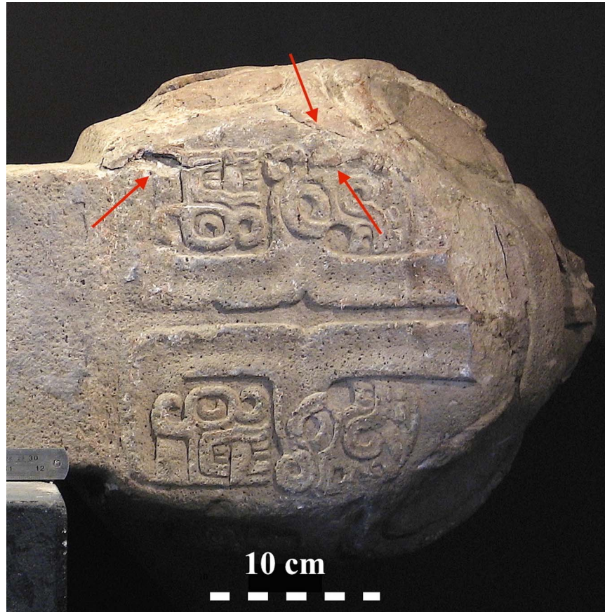
FIGURE 4. Hair cracks and cracks in ID16. It can be seen how the hair cracks (right to left) produce the detachment of polished cortex.
