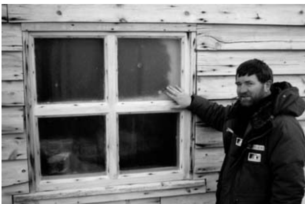
Fig. 13. Abraded glass of window on southeast wall, Scott's hut Cape Evans. January 1998.
