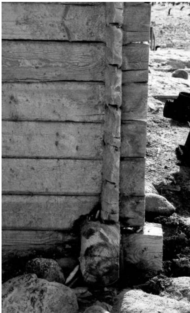
Fig. 4. Weathered northeast corner, Borchgrevink's 'stores hut' with coating of salt and sand particles. January 2003.
