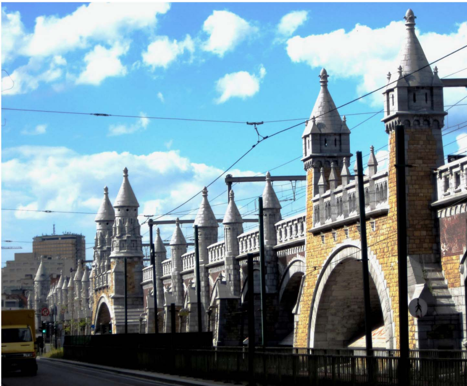
Figure 4. Railway overpass in the Antwerp Zurenborg district.
