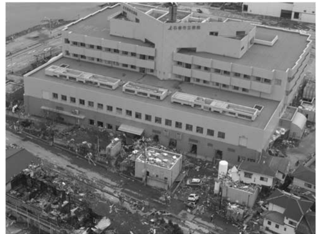
Figure 2. The tsunami destroyed the first and second floor of Ishinomaki Municipal Hospital.
