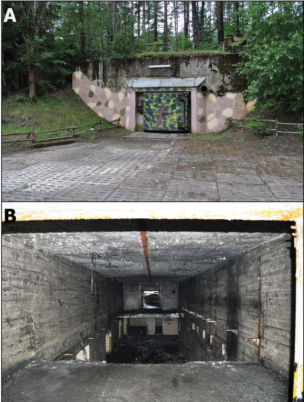
Figure 3. A) Monolit bunker in Podborsko, preserved in its original condition. The facade exhibits a modern fluorescent lamp and a recent failed attempt to reconstruct the camouflage pattern; B) the plundered interior of the Monolit bunker in Brzeznica Kolonia (photographs by G. Kiarszys).
