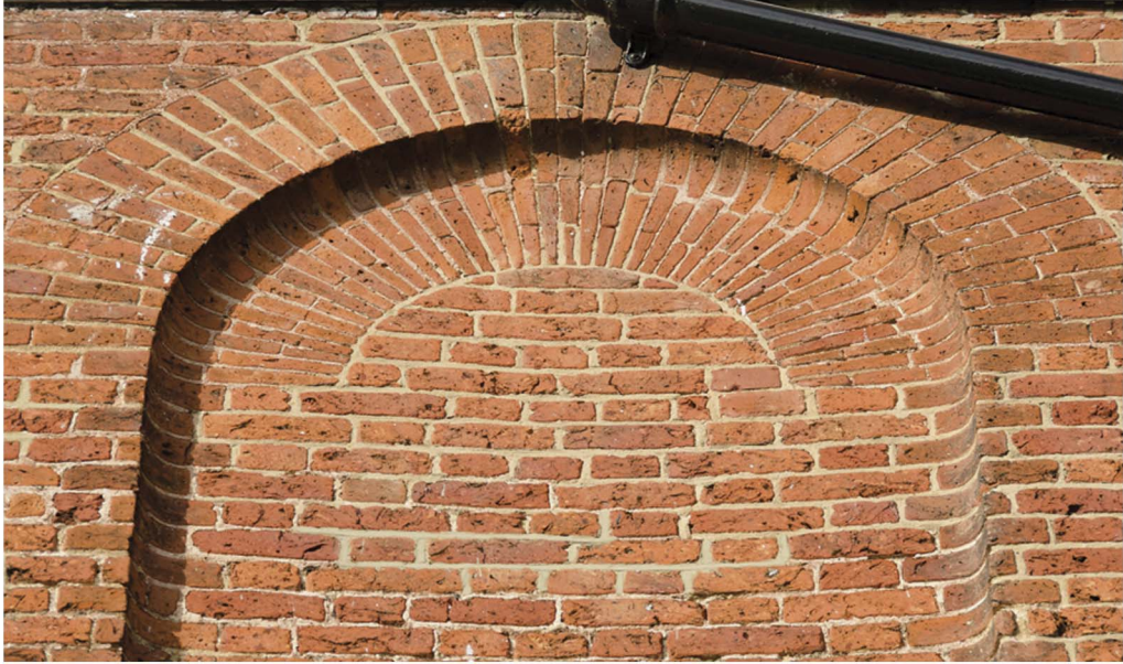
Fig 19. Eltham Lodge: detail of brick recess on south front with concave reveals.
