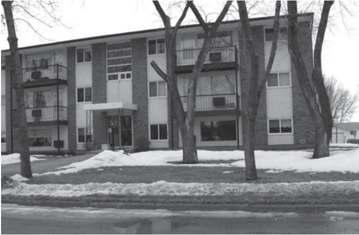
Figure 2. 'Very unfriendly to seniors. Bottom apartments are eight steps down. Second floor eight steps up, and third floor 24 or more steps up. No elevator: difficult access for seniors. Impossible access for those confined to wheelchairs. This town has numerous apartments constructed to these standards.'
