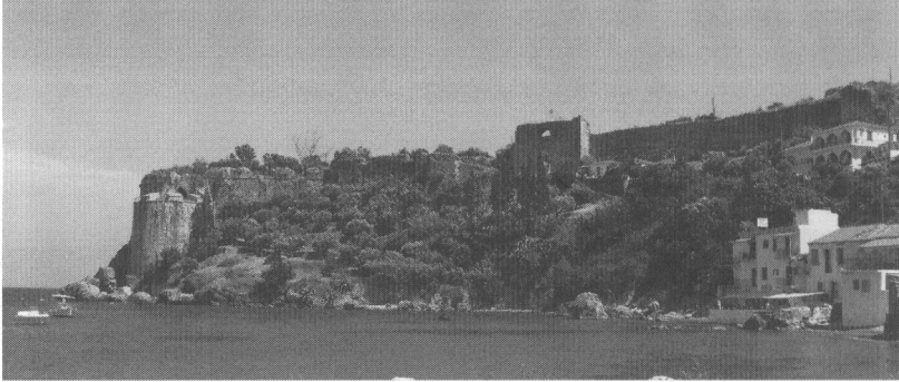
Fig. 8. The north side of the walls with the Twin Bastion (left) and the Main Gate (centre) (N. Kontogiannis).
