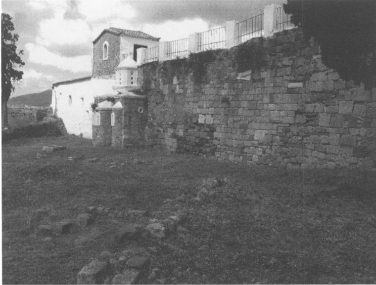
Fig. 6. Transversal Wall, exterior view (I. Grigoropoulou).
