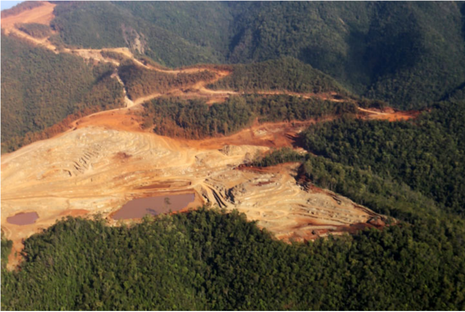
Figure 3. Rupture, The Maracuan Nickel Mine. Source: Jonah Van Beijnen.
