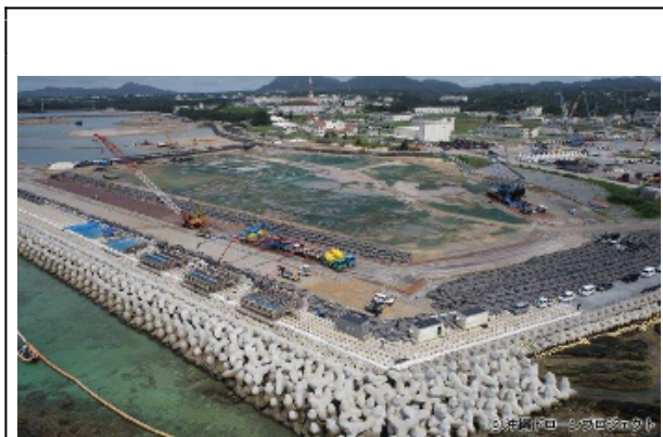
Construction work on the Henoko-side (July 2020).
