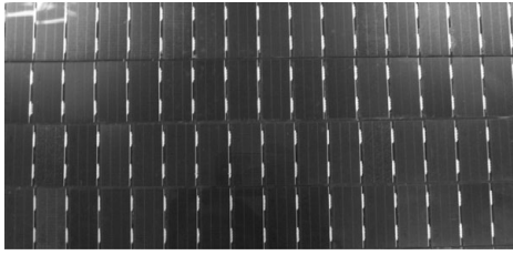
Fig. 15. Photograph of a solar array constructed in the auto-laydown method.
