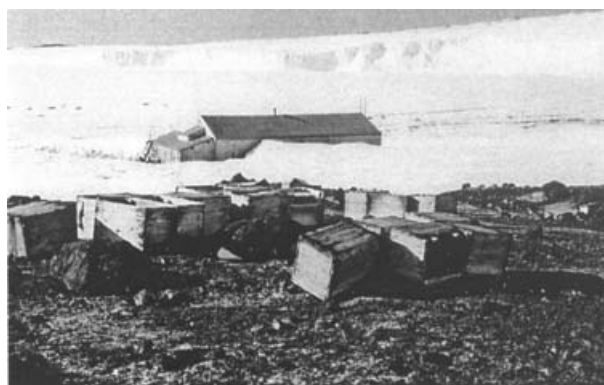
Fig. 1. Fuel depot at Cape Evans near the historic hut. High concentrations of polyaromatic hydrocarbons are in soils below and around the fuel containers.
