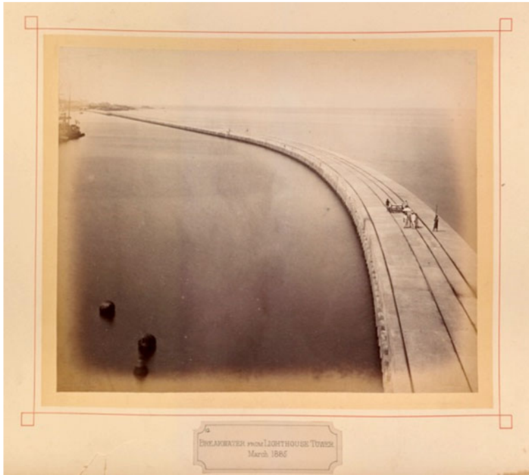
FIGURE 13 “Breakwater from Lighthouse Tower, March 1885,” “Colombo Harbour, Completed, 1885.” Source: GBR/0115/Y303C, Royal Commonwealth Society Collections, Cambridge University Library.
