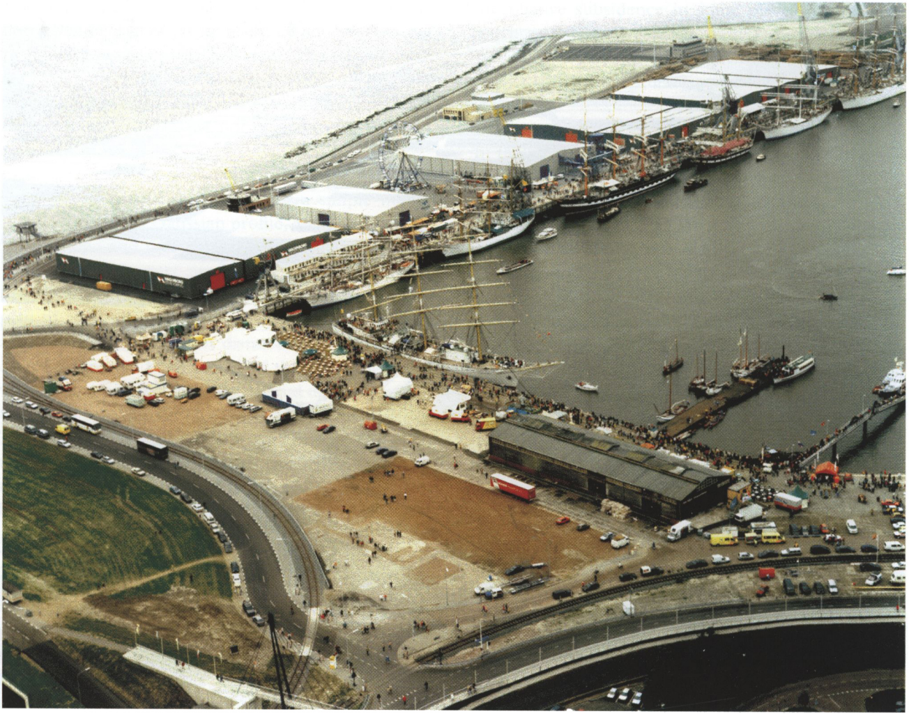
Fig. 9. Photograph of the port of Delfzijl (Luchtfoto Aerophoto Eelde).
