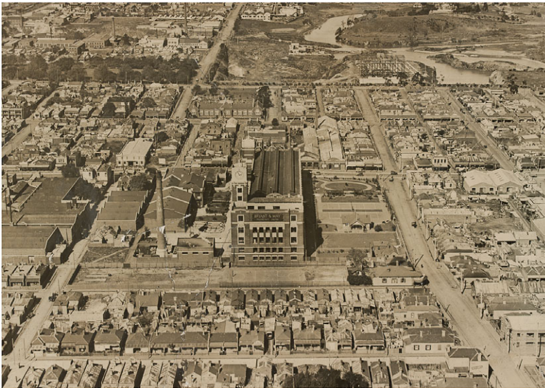
Figure 1. Aerial view of the Bryant & May factory in Melbourne, looking east from Green St. Richmond, the Yarra River in the background.
