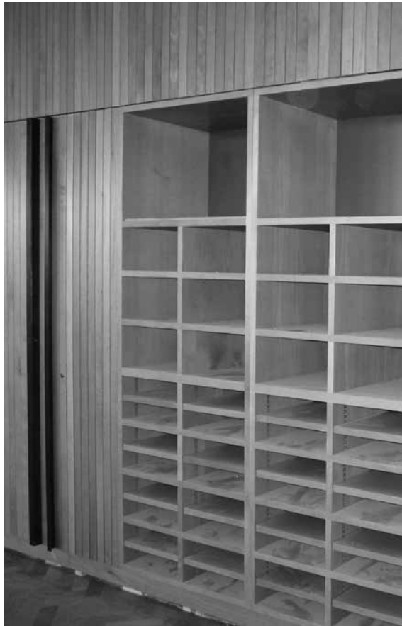
11 Joinery details. The joinery softens the hard surfaces on every floor of the Tower and allows for much needed storage and sink units in the studios and pigeonholes in the reception area shown here.
