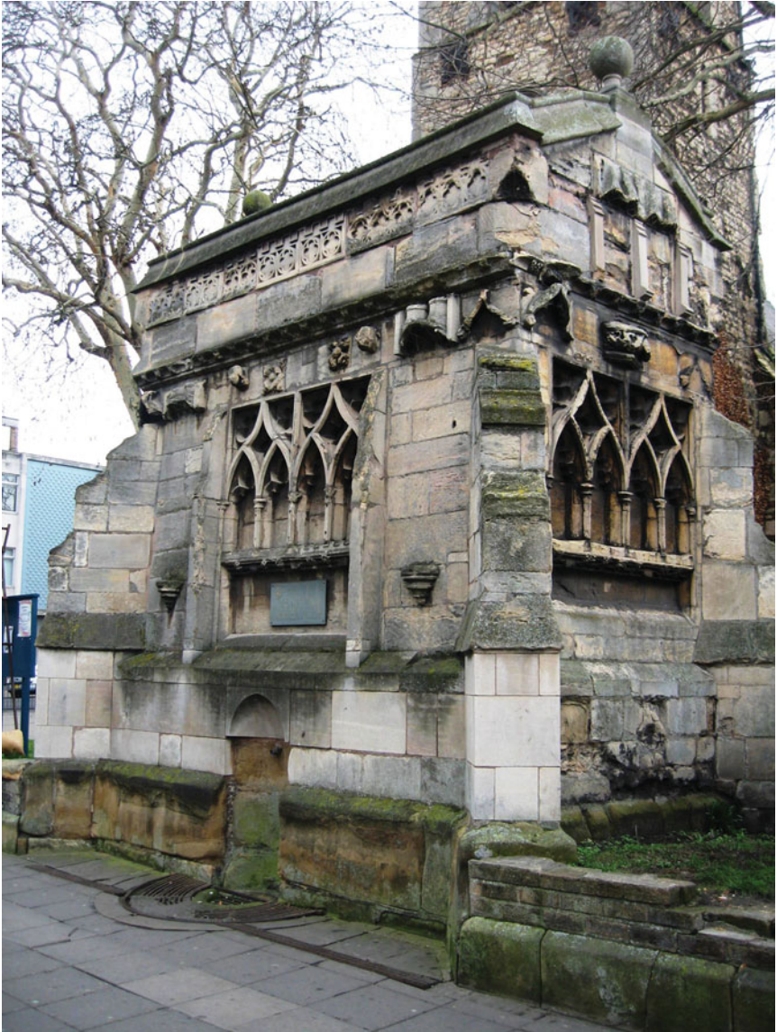
Figure 2: (Colour online) Conduit house at St Mary-le-Wigford, Lincoln, erected 1540 and re-using masonry fragments, probably from the Carmelite friary. Originally sited in the High Street, it was moved into a nearby churchyard in 1864.
