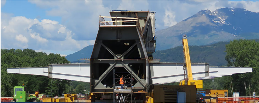
Figure 1. Main beam of the Marchetti bridge (Chiaia et al., 2019) Springer Nature Switzerland AG 2020. This figure has been reproduced with the permission of the copyright holder, and is not included in the Creative Commons licence applied to this article. For other re-use, please contact the copyright holder.
