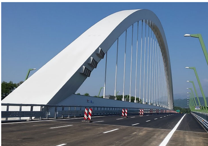
Figure 2. Arch of the Marchetti bridge (Chiaia et al., 2019) Springer Nature Switzerland AG 2020. This figure has been reproduced with the permission of the copyright holder, and is not included in the Creative Commons licence applied to this article. For other re-use, please contact the copyright holder.
