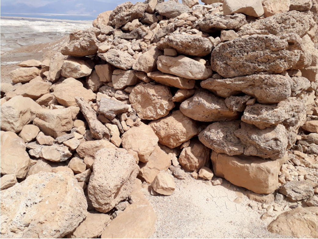
Fig. 7. Tower 10 and the wall abutting it (view to the east). (Photograph by H. Ashkenazi.)
