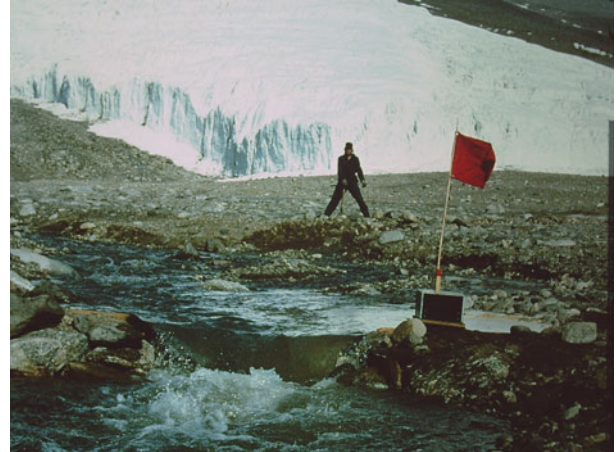
Fig. 66. 1984–1985. The Bartley east weir at near maximum capacity.
