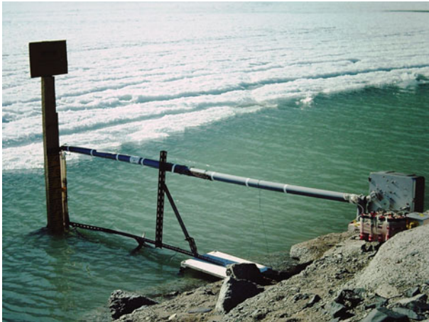
Fig. 68. 1983–1984. The Lake Vanda surface-follower recorder installation.
