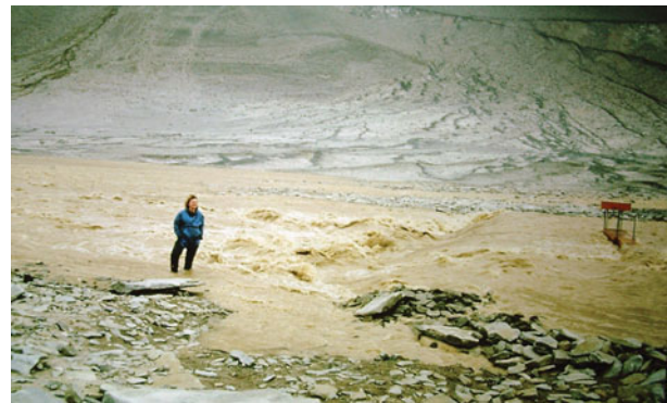
Fig. 80. 1986–1987. The weir and water level recorder during the January flood (Photo. C. Lynch).
