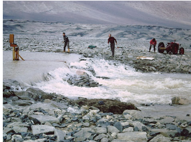
Fig. 12. 1970–1971. Alarmed by the first weir overflow, the Vanda staff were co-opted into the ‘save-the-weir’ emergency rock tossing.
