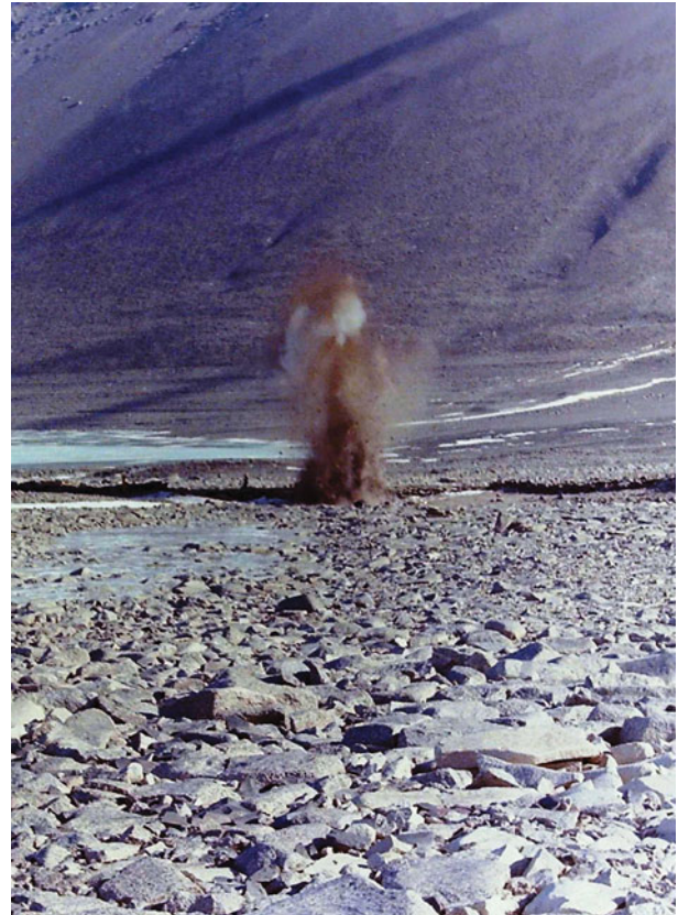
Fig. 75. 1985–1986. The new weir excavation was assisted by explosives.
