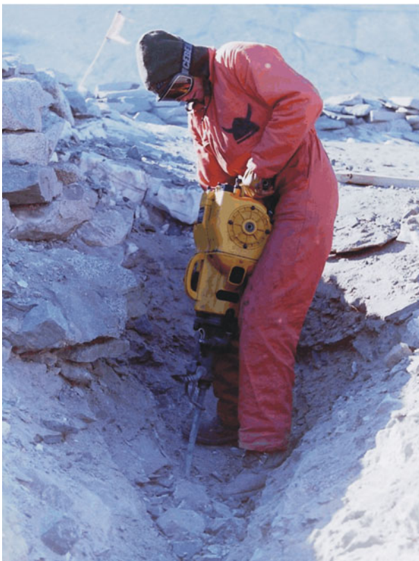
Fig. 74. 1985–1986. Mason excavating the new weir trench by jack-hammer.
