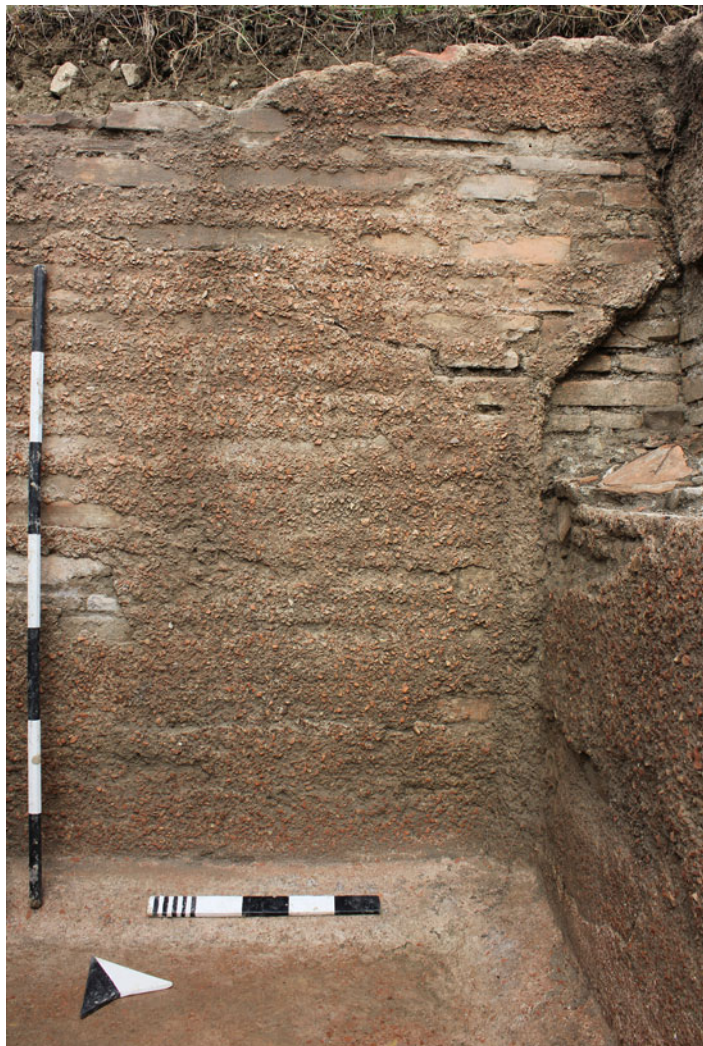
Fig. 2. The northern internal wall of the cistern (Area 3).
