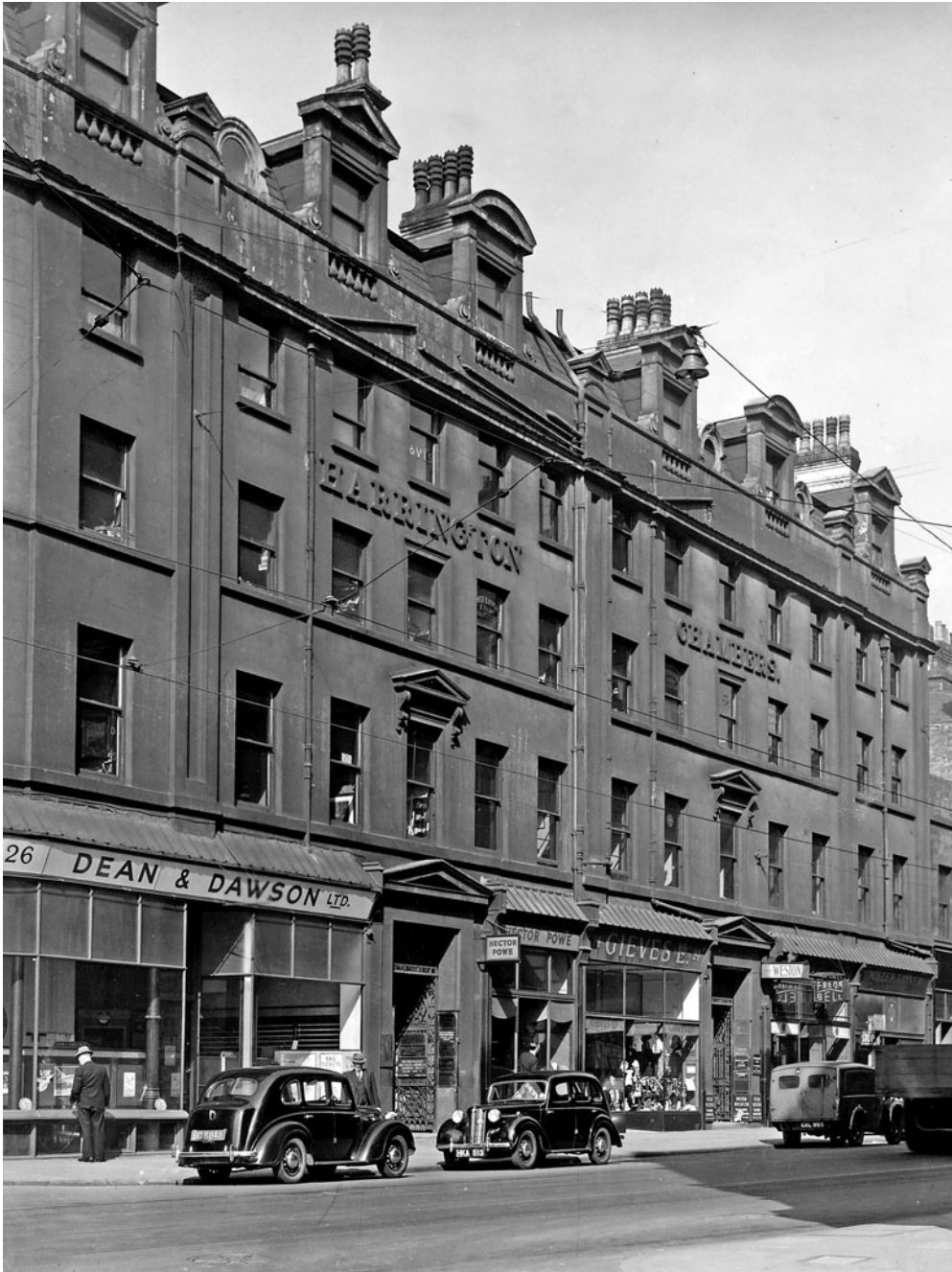
Fig. 5. Harrington Chambers, built about 1830, photographed in 1948. The pedimented dormers and projecting shop fronts appear to be late nineteenth-century alterations (Liverpool Record Office, Liverpool Libraries, CE 8926)
