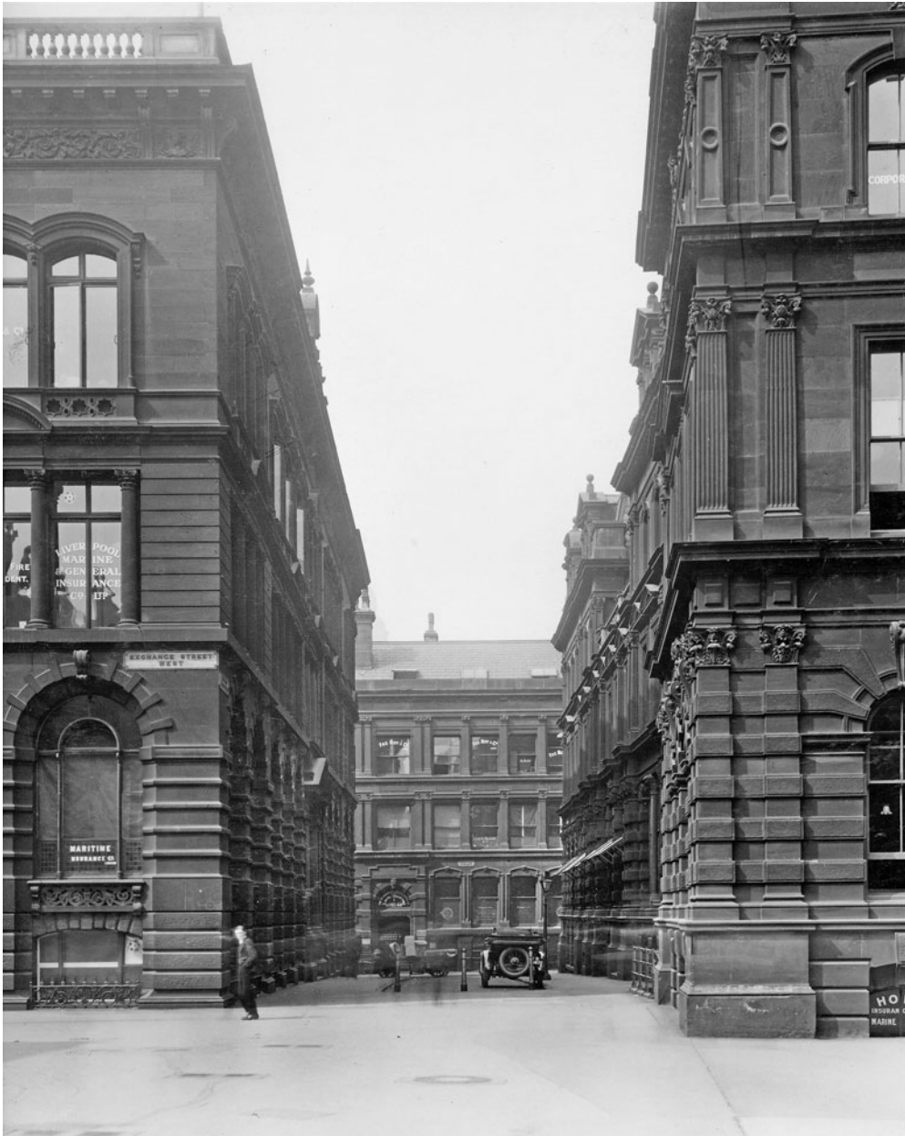
Fig. 20. Exchange Passage West, photographed by Stewart Bale c. 1922. Brown's Buildings is on the left, Exchange Buildings on the right, Borough Buildings straight ahead (Liverpool Record Office, Liverpool Libraries, Acc. 4647)
