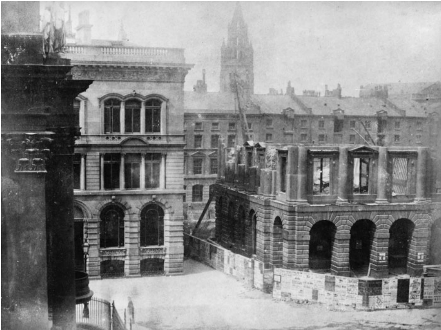
Fig. 10. Demolition of the Wyatt-Foster Exchange Buildings in 1864. The Corinthian order of the Town Hall is in the left foreground, with the clean new stonework of Brown's Buildings behind. The warehouses in the background were replaced by Peters' Buildings soon after this photograph was taken — see Fig. 17 (Historic England Archive)
