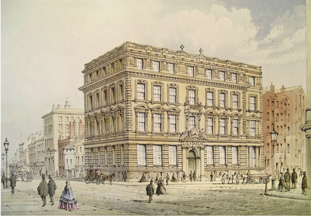
Fig. 13. Royal Insurance Buildings, 1848, by William Grellier, from William Herdman, Views in Modern Liverpool, 1864, pl. 24, opp. p. 32 (Liverpool Record Office, Liverpool Libraries)
