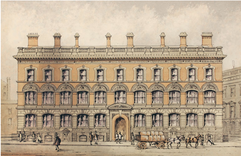
Fig. 12. Albany Building, 1856–58, by J.K. Colling, from William Herdman, Views in Modern Liverpool, 1864, pl. 39, opp. p. 49. The width of the windows in proportion to their height is striking (Liverpool Record Office, Liverpool Libraries)
