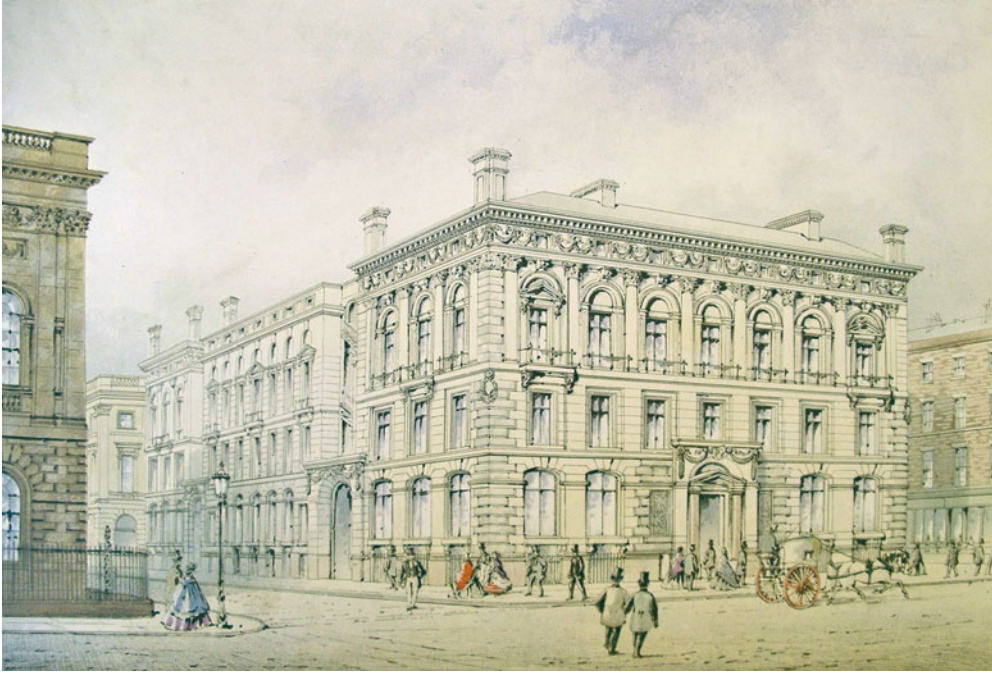
Fig. 11. Liverpool & London Chambers, 1856–58, by C.R. Cockerell, from William Herdman, Views in Modern Liverpool, 1864, pl. 25, opp. p. 33. The front block contained the company's offices, with three blocks of speculative offices behind, linked by bays containing stairs and entrances (Liverpool Record Office, Liverpool Libraries)
