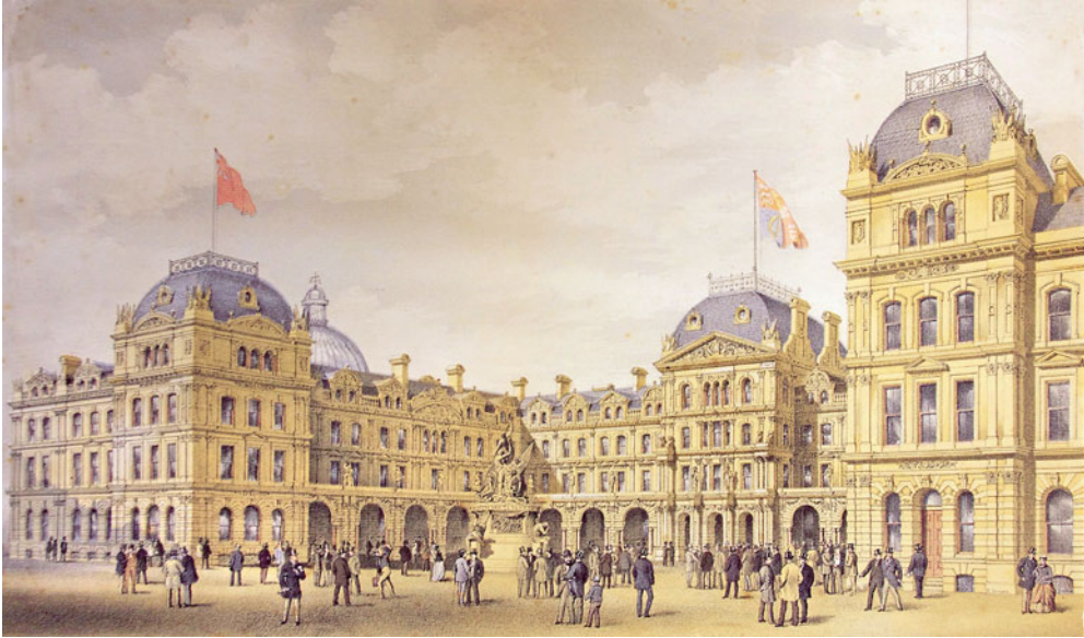
Fig. 9. The Exchange Buildings of 1863–70 by T.H. Wyatt, in a lithograph of 1865. The arcades are single-storey projections, preserving a hallowed feature of the previous Exchange Buildings without using valuable ground-floor office space (Liverpool Record Office, Liverpool Libraries, Hf 942.7213 EXC)
