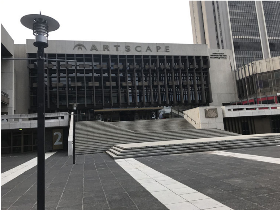
Figure 8. Front entrance of Artscape, formerly the Nico Malan, with the Civic Centre's administrative wing visible to the right of the image. (colour online)
