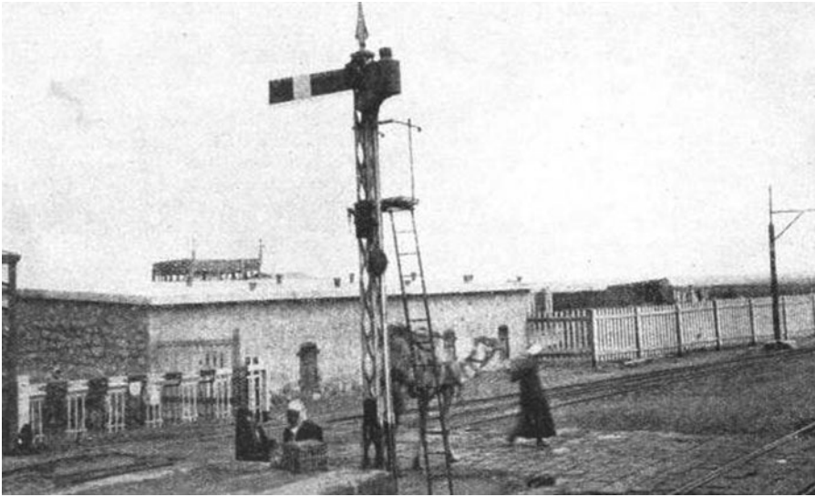
Figure 1. A rail crossing with mechanical signaling in Egypt, ca. 1930. Source: “In the Nile Valley: Train Operation in Modern Egypt,” Railway Wonders of the World 2 , part 41 (1935): 1314.
