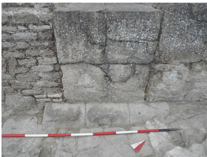
Fig. 7. Tufo pilaster (SU 5755) with moulded base, abutted by slab pavement, at the southern limit of ROOM F 1 -3.
