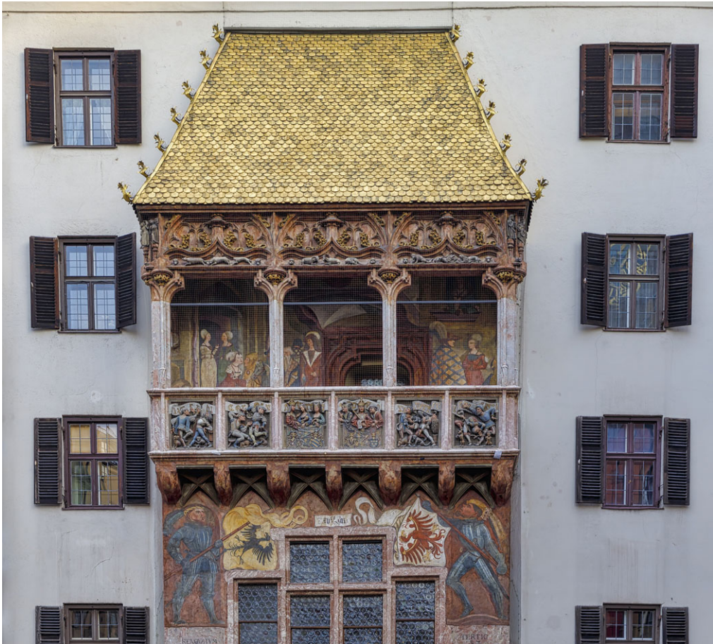
Fig 5. The Goldenes Dachl, Innsbruck, 1498–1500. The roof is covered with fire-gilded copper tiles and may be similar in appearance to the covering of ‘white plate scallape wise’ recorded on the timber lodging used at Boulogne in 1544. Photograph : © Laszlo Szirtesi/Getty Images.
