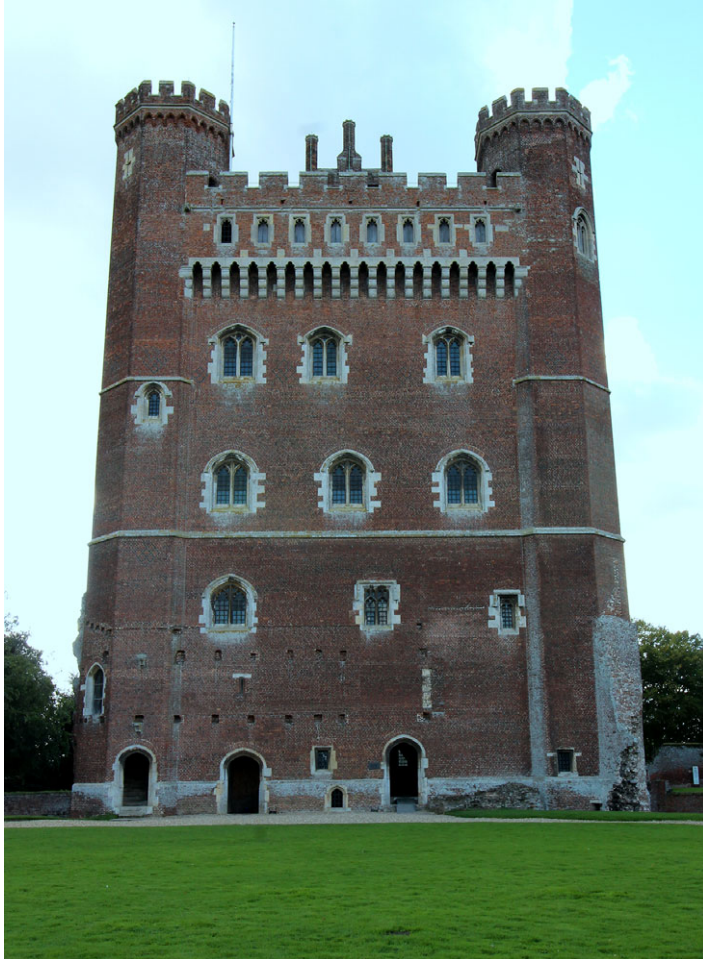
Fig 7. East elevation of the great tower. Photograph: the author.
