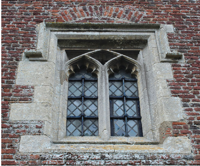
Fig 21. Window tracery of the Middle Ward lodgings. Photograph: the author.
