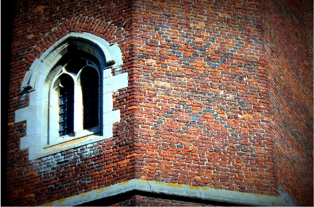
Fig 12. M and double-V designs picked out in the diaperwork of the south-west turret. Photograph: the author.
