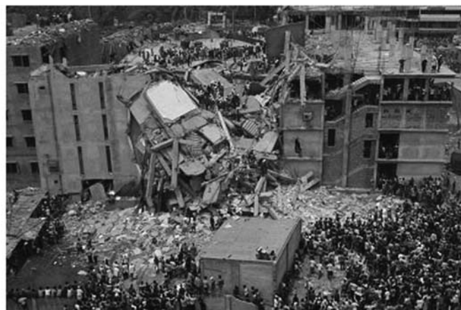
Aerial view of the building following the disaster
