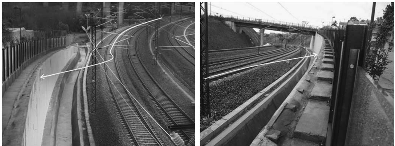
Figure 2. The Curve from Different Directions Where the Train Set Derailed. Observe the sharp edge of the water chute (right). (Photo: Rebecca Forsberg).
