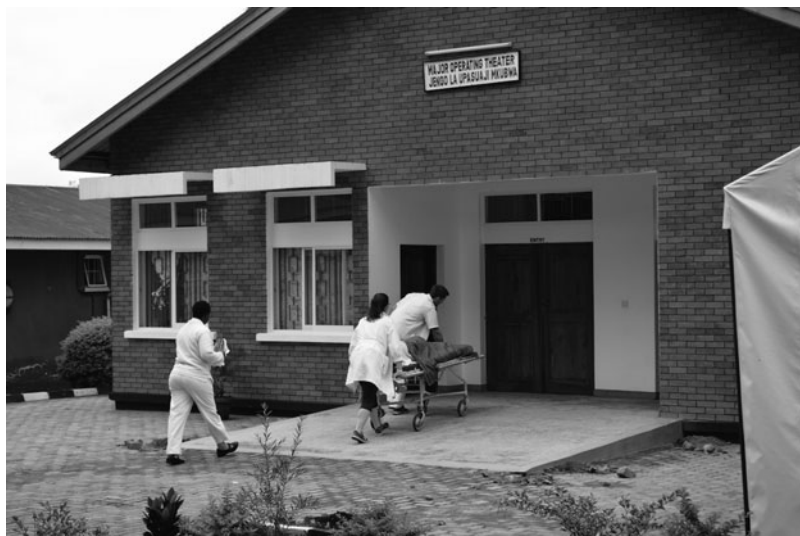
FIGURE 2 Two foreign volunteers and the head surgical nurse enter the newly completed major operating theatre of Kiunga District Hospital with a patient, 24 June 2014.
