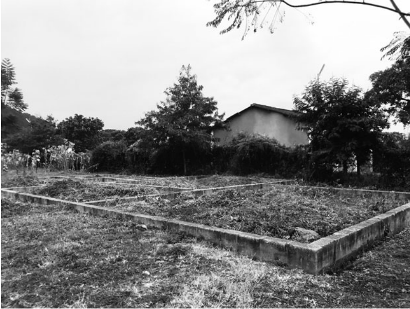
FIGURE 3 Foundations of the since abandoned modern mortuary project at Kiunga District Hospital, 27 July 2017.
