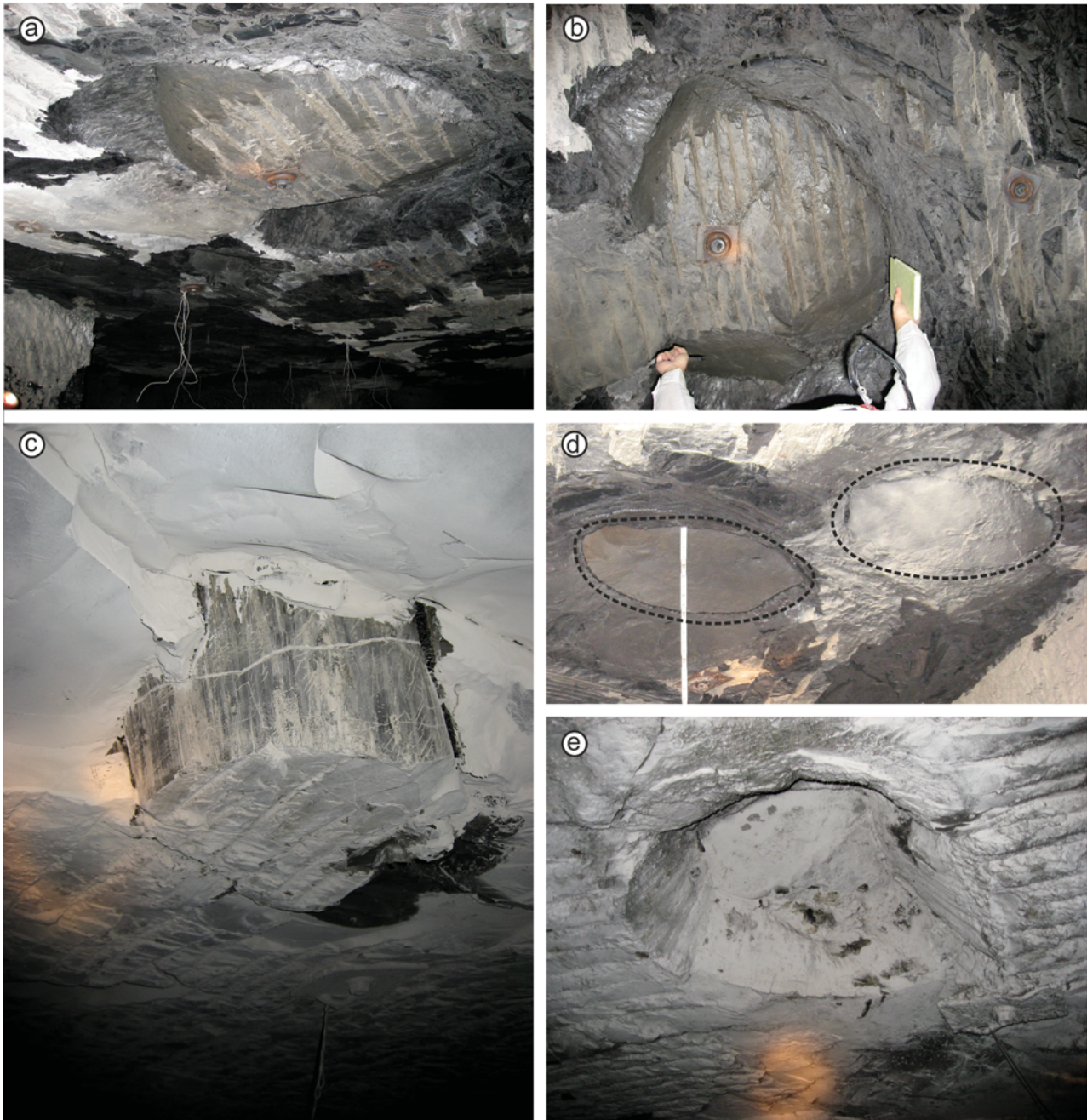
Figure 15. (Colour online) Large fossilized plant remains can be hazardous structures in coal mines, in particular kettle bottoms which are stumps that are slickensided and liable to fall out of the mine roof. Examples from the Springfield (No. 5) Coal (late Desmoinesian age, early Cantabrian, Middle Pennsylvanian), USA (all photographs courtesy of Dr W. A. DiMichele): (a, b) a bolted stump in the roof of the Prosperity Mine, Illinois, (a) looking along the gallery and; (b) looking directly up at the stump in the roof (both photographs taken in 2007); (c) a tree trunk protrudes from the roof of the Galatia North Mine (2006); (d) two in situ kettle bottoms (inside dashed ellipses) side by side in the roof of a mine in Indiana (note the thin coalified layer surrounding each stump base, just inside dashed ellipses); and (e) space left after a kettle bottom has come out of the roof of the Galatia North Mine, Illinois (2006).
