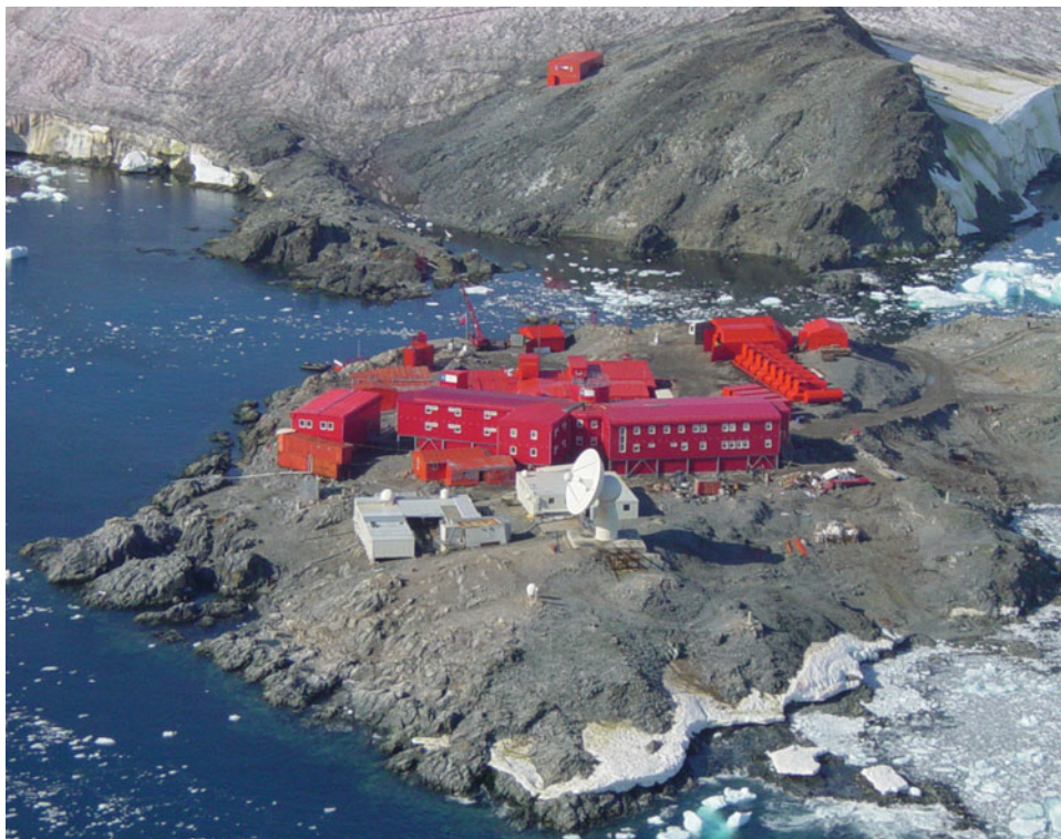
Fig. 2. (Colour online) Aerial view of the Antarctic base Bernardo O'Higgins with the German facilities (white buildings) in front (photo: M. Specht).
