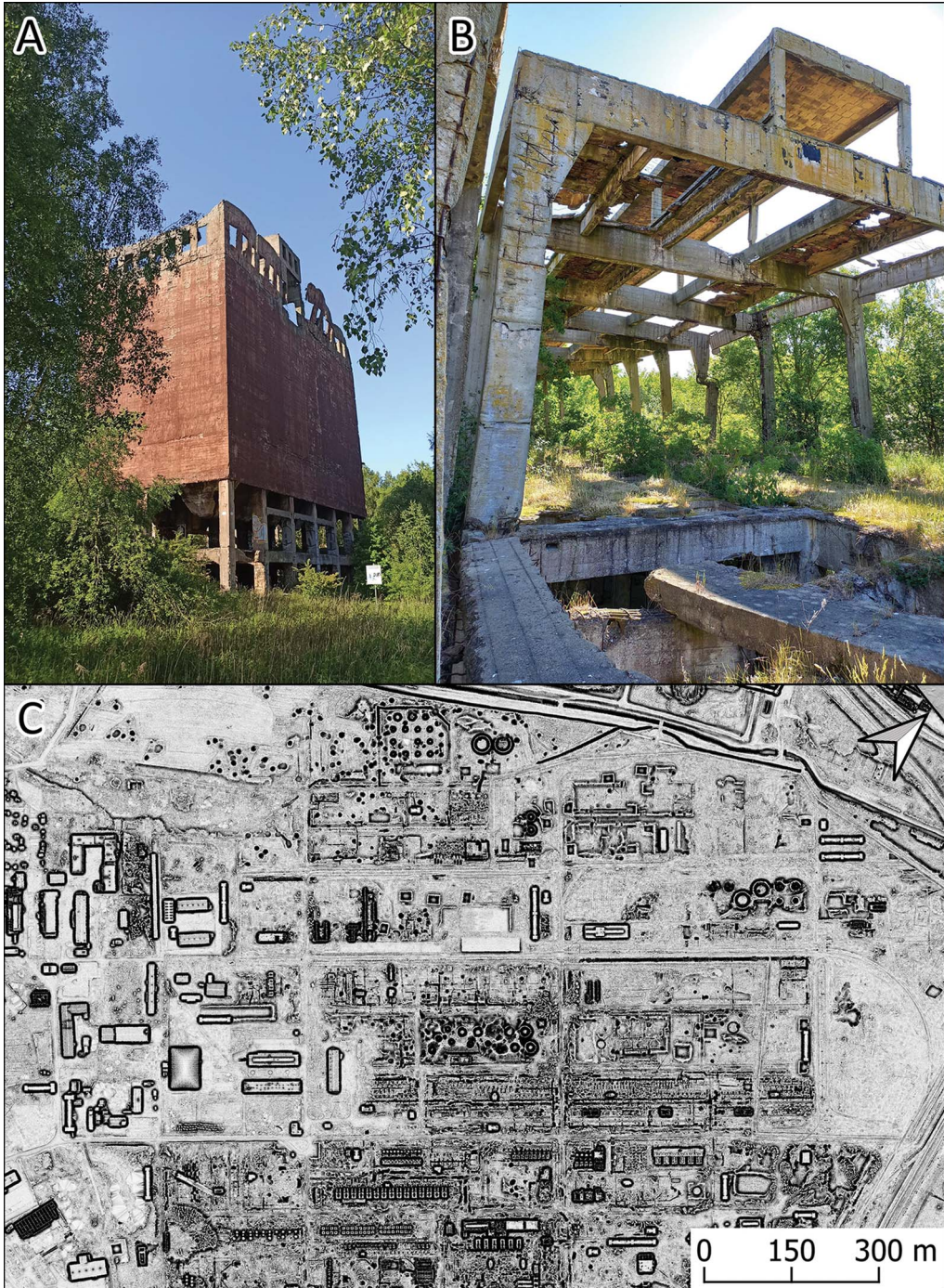
Figure 8. The ruins of the plant: A) the multi-storey coal mill; B) the concrete frame of the coal power plant; C) preserved relics of the plant registered by ALS (openness-positive) (figure by G. Kiarszys).
