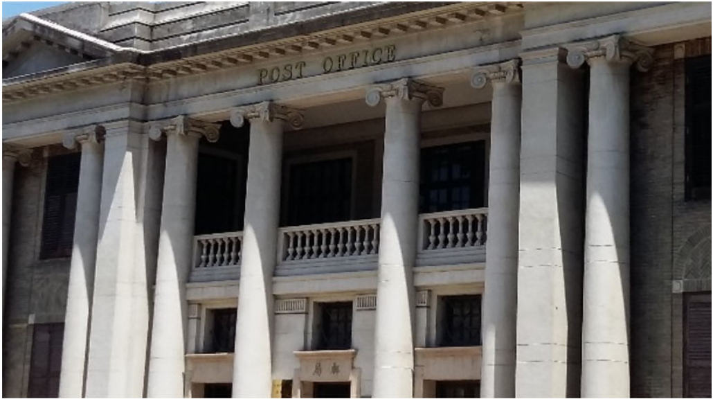
Figure 5. The old central post office in Shantou
